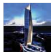
Al Hamra Tower - Kuwait
