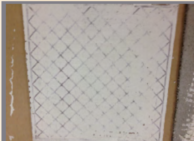
A properly back buttered large format tile.
