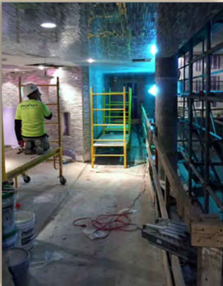
Photo Courtesy of Profast Commercial Flooring
