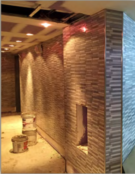
Photo Courtesy of Profast Commercial Flooring
